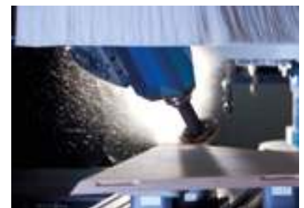
Trimming of inclined grooves for panel connection
