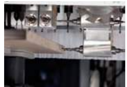
Horizontal boreholes for carcass connections
