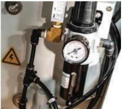
• Regulator, filter and primary shut off value for easy pneumatic connection.
